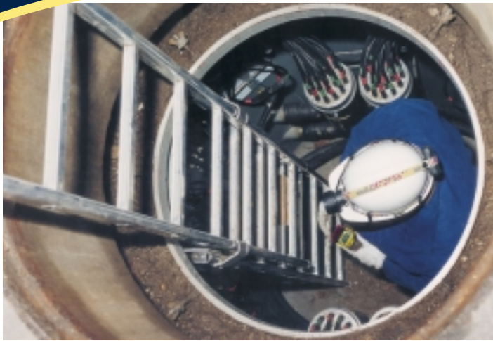
Example of application : operation in confined area
